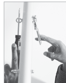
Figure 9: Use two fingers to tighten bolts
